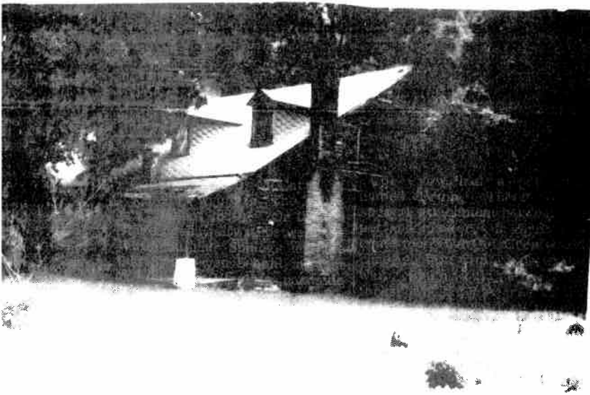
CROWS—West elevation, showing three of the large brick chimneys and a small one which seems to be of more recent construction.
